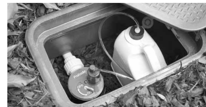
Figure 5: A properly installed ProFeeder will look something like the illustration above. Notice that the valve box has been placed in the opposite direction of the irrigation system piping to make plenty of room for the fertilizer bottle. A jumbo valve box may also be used to accommodate larger fertilizer bottles for larger landscapes.
